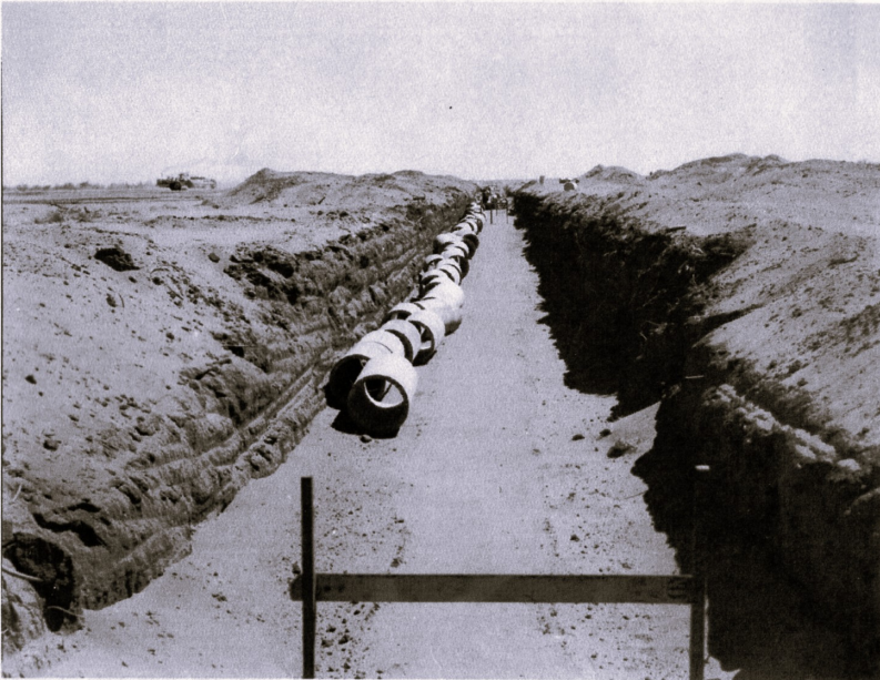
[above] Drainage lines being installed to the airstrip with leveling machinery at work in top left of image; [below] on ground water tank under construction with bore to right. Source: National Archives of Australia.
